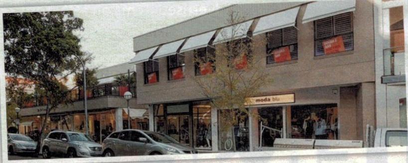
Existing buildings at 20-26 Cross St, Double Bay.
